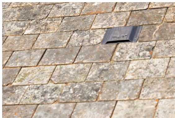
20 Nov 25 – Bat entrances built into the roof.
