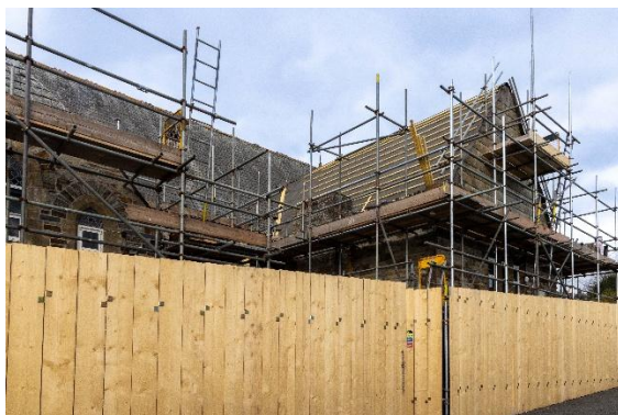
1 Oct 25 - Haras fencing and south scaffolding
