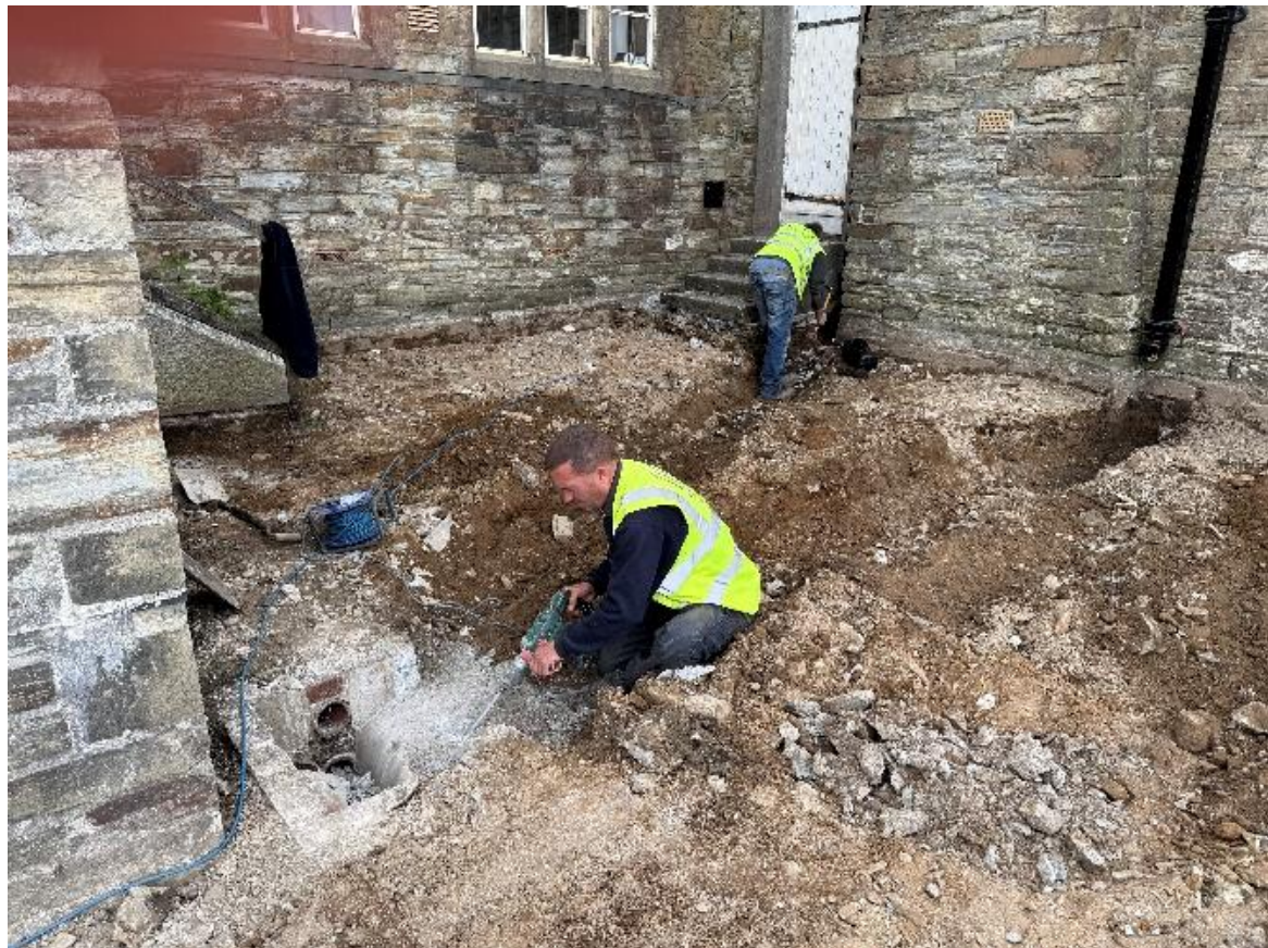
28 Apr 26 – preparing the new channels for the drains.
