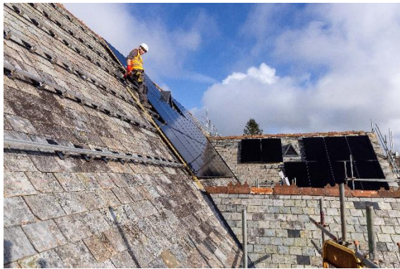
6 Feb 26 – Solar panels being installed
