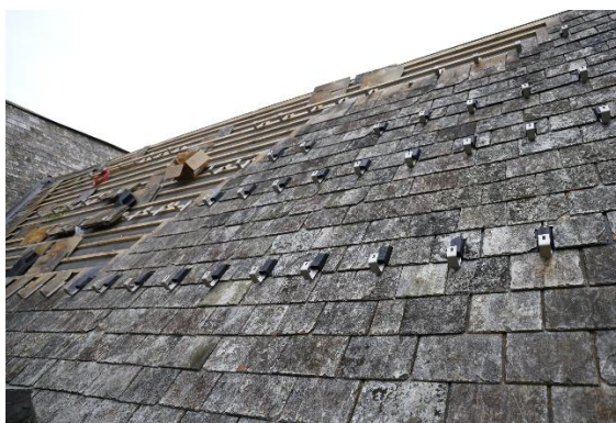
26 Nov 25 – Solar panel hooks in place for grid
