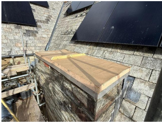
12 Feb 26 – remove the old capping and build new frame.
