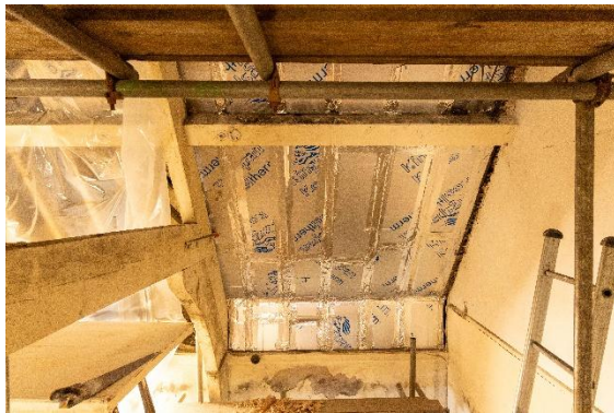
4 Feb 26 – New insulated plasterboard ceiling in the inner lobby area
