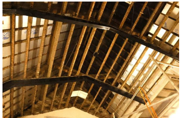
12 Jan 26 – Old plasterboard ceilings removed
