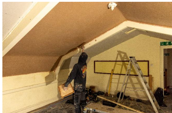
26 Nov 25 –plastering over new insulated ceiling in upstairs room, the "Upper Room".
