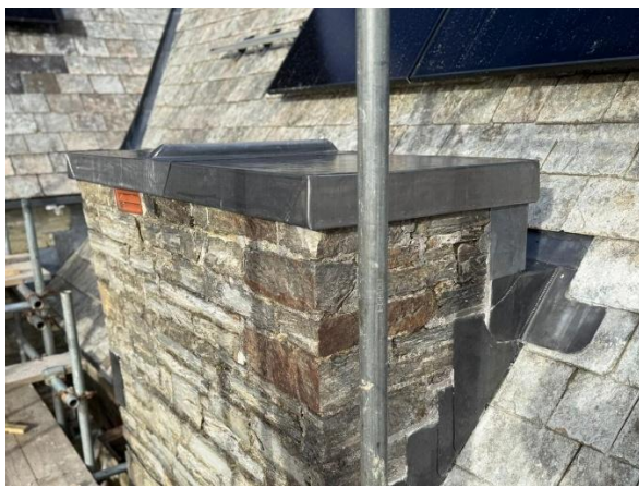
12 Feb 26 – the new lead capping is finished.
