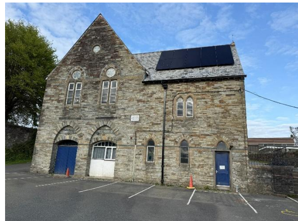
20 Apr 26 – Solar panels on the rear west-facing roof slope.
