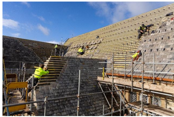
20 Nov 25 – reroofing the south roof around the solar panel hooks
