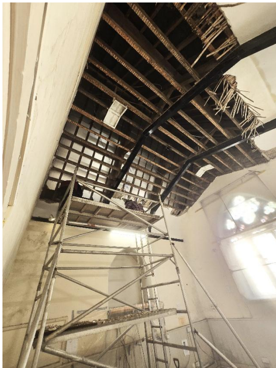
6 Jan 26 – Work begins in the church office.
