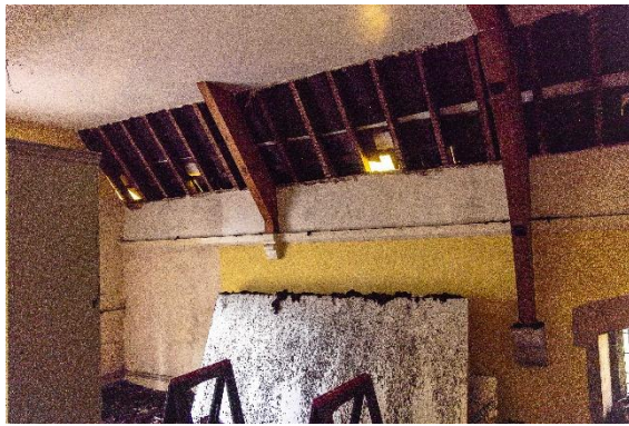
26 Nov 25 – Removing old plasterboard ceiling in upstairs room "Siloam"
