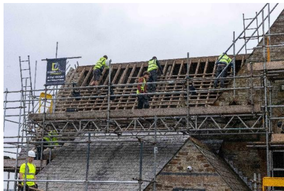
14 Oct 25 – The roofers arrive and start stripping the front east-facing roof
