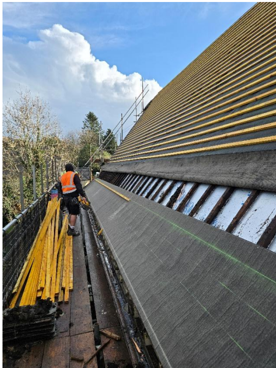
2 Dec 25 – Felt and battening after insulation added in-between the roof rafters.
