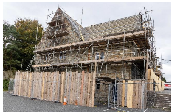
1 Oct 25 - Haras fencing and west scaffolding
