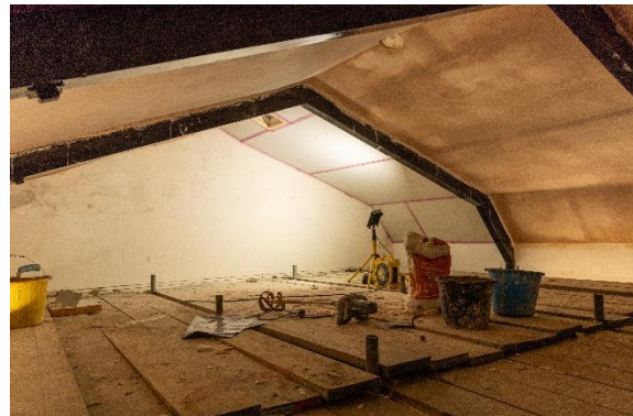
4 Feb 26 – New insulated plasterboard ceiling being plastered in the "Upper Room"
