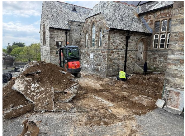
28 Apr 26 – digging up the old concrete.
