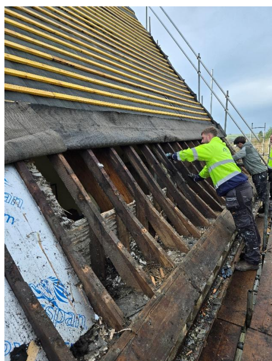
2 Dec 25 – Preparations before adding the final insulation to the north roof.
