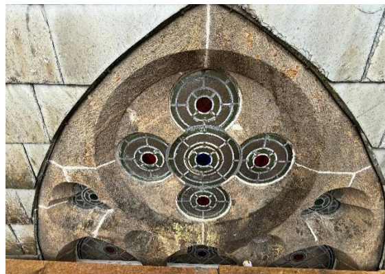
27 Mar 26 – repointing completed around the oriel windows
