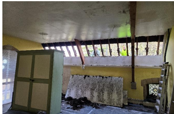
2 Dec 2025 – Roof stripped outside "Siloam", ready for the insulation.
