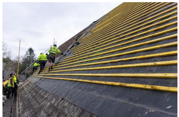
26 Nov 25 – Stripping slates, insulating, then felting and battening the north roof.
