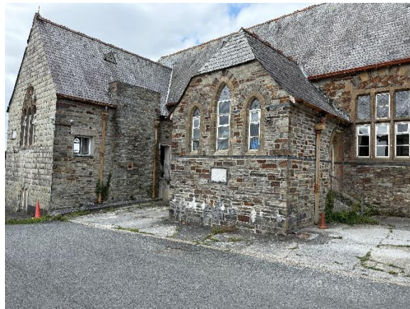
21 Aug 25 – the starting point, with all the cracked and broken concrete.
