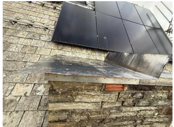
12 Feb 26 – start covering the new frame with lead.
