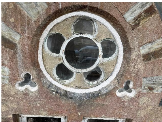
27 Mar 26 – repointing completed and external secondary glazing fitted.
