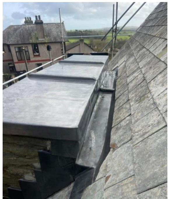
12 Feb 26 – the second, larger chimney is also finished.
