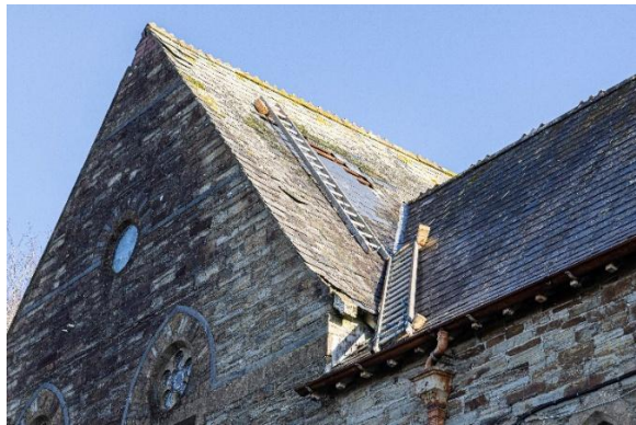
Emergency repair work to roof following Storm Henk.
