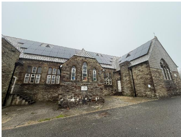
20 Apr 26 – Solar panels on the south and west roof slopes
