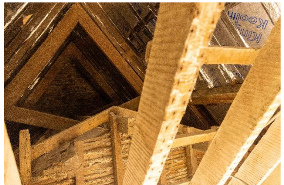
4 Feb 26 – Insulation between the roof rafters
